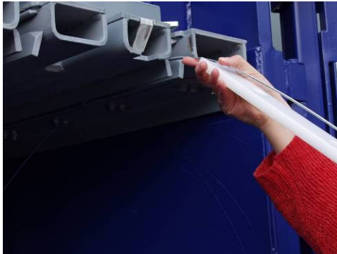
Bild 5-4 Attaching the wire pulling hook
